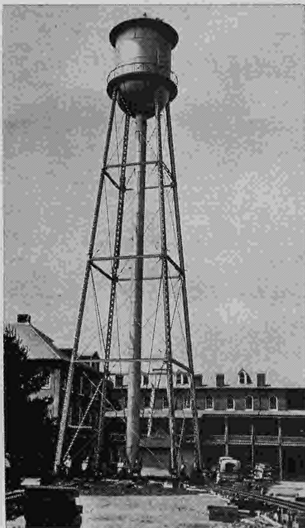
MOVING OF THE WATER TOWER AT CONVENT
